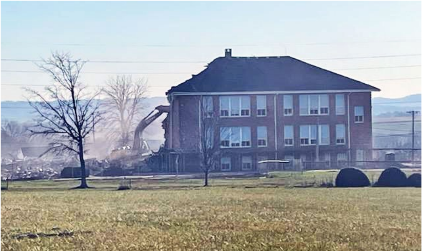
The original building was the last to go.
