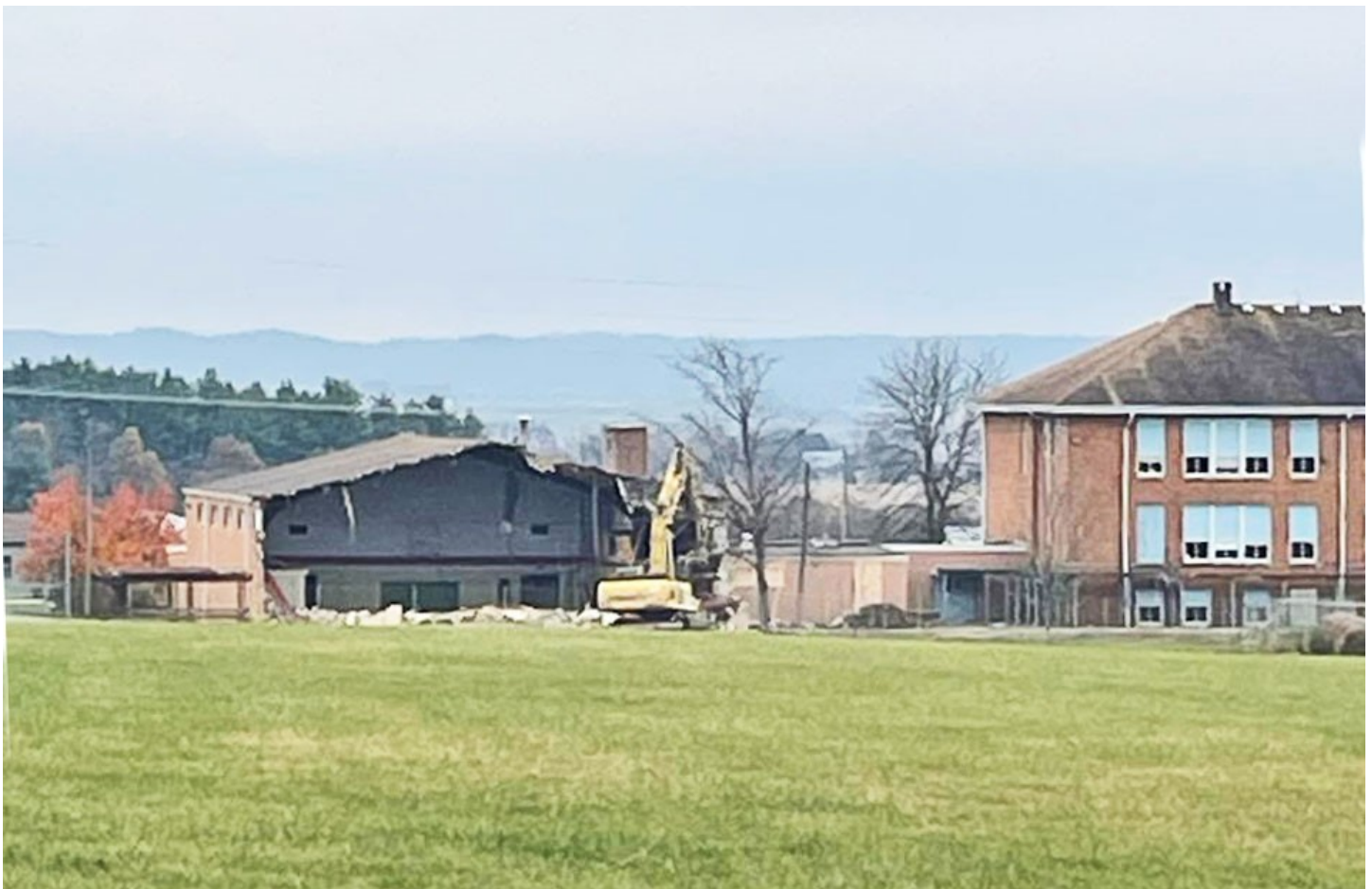
The gymnasium was the first to be demolished
